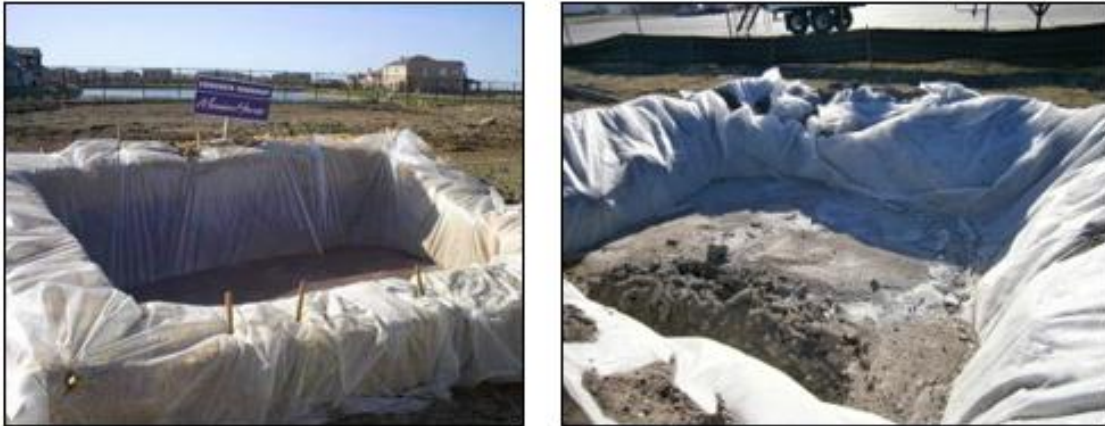
Plate 3-1 Typical concrete wash out areas
